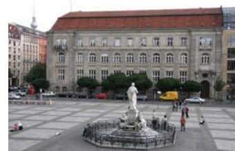
View to the building of the Berlin-Brandenburg Academy of Sciences
